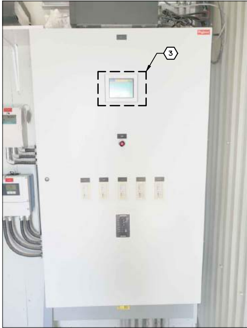
MAIN LIFT STATION CONTROL PANEL EXTERIOR DEMOLITION
