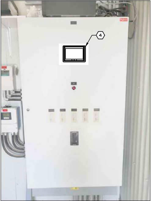
MAIN LIFT STATION CONTROL PANEL EXTERIOR PROPOSED
