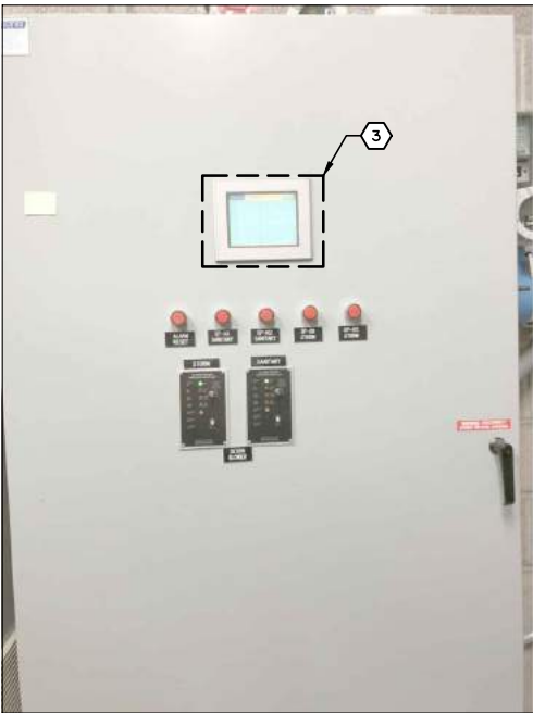
SUNDANCE RIDGE LIFT STATION CONTROL PANEL EXTERIOR DEMOLITION NTS
